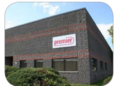
Premier's state-of-the-art instrument plant is located in Philadelphia, PA USA.
